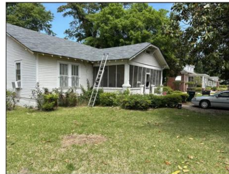
1.0 New Roof covering installed.
